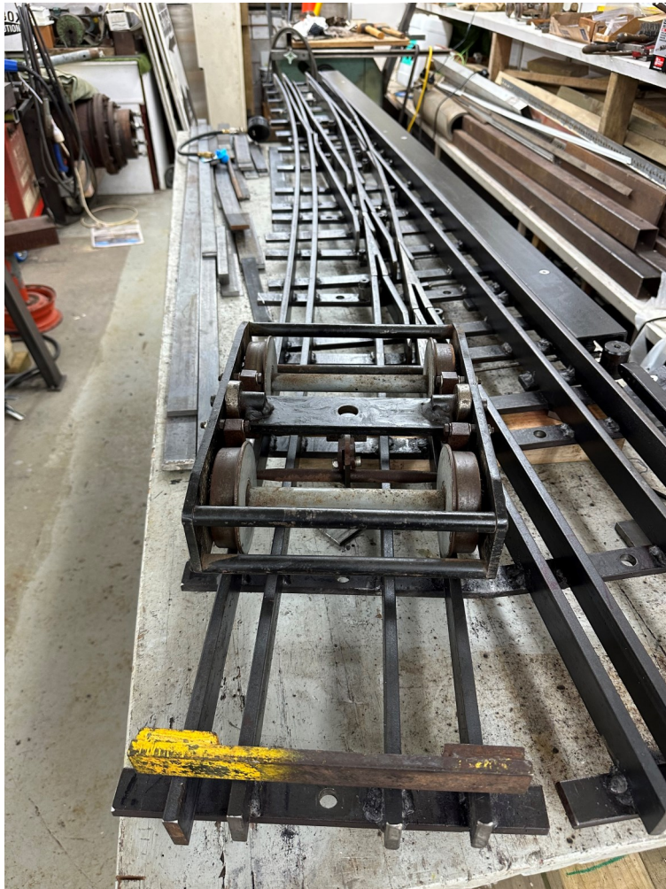
Points construction in progress...
