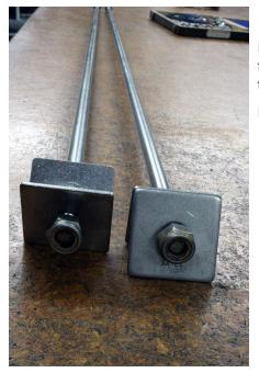
New tie bars for the back steps by the clubrooms are made from Stainless Steel and should long outlast the original ones that had all but rusted through.
